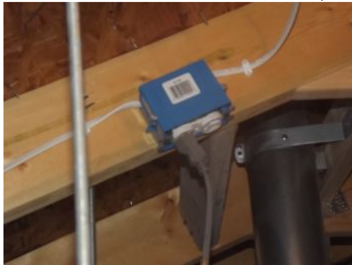
Outlets in single car garage were not functional, should be GFCI when functional, recommend correction by licensed professional
