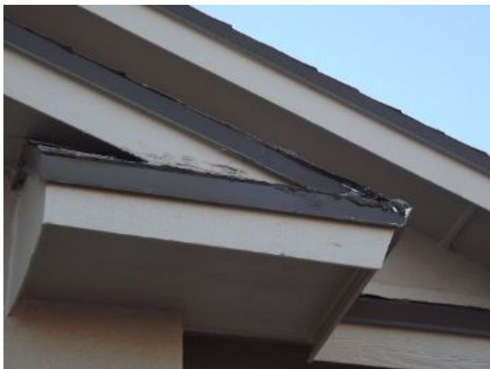
Certain areas of roof were unsealed, or needed more weather proofing via tar and granulars, recommend correction by licensed professional
