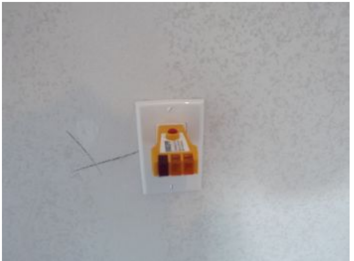
Outlets in single car garage were not functional, should be GFCI when functional, recommend correction by licensed professional
